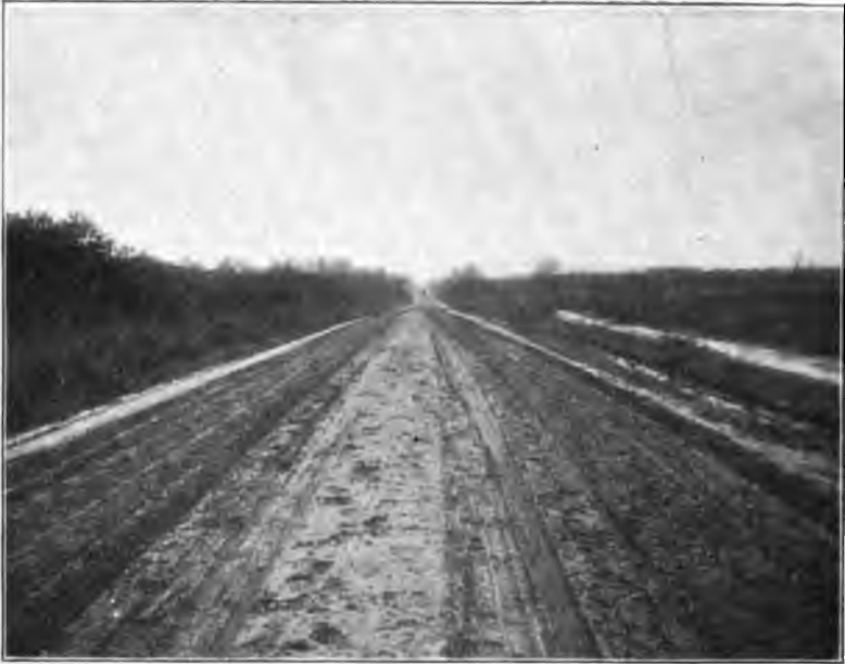
Corliss Avenue, Monmouth Co., before improvement.
